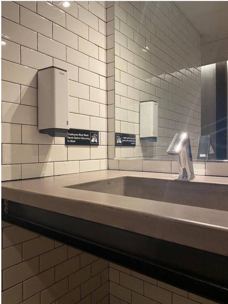
Rail Haus' ADA rest rooms include sinks that allow clear floor space and grab bars surrounding toilets.
